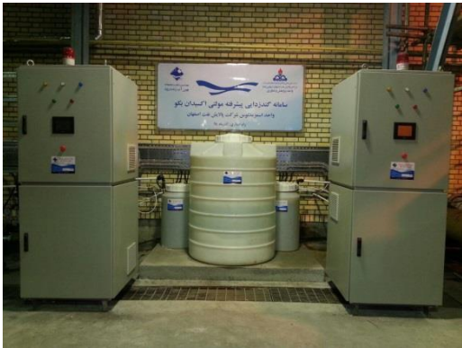
Industrial Water Disinfection Plant RO Plant - Esfahan Oil Refining Co.-Esfahan -2020 Capacity: 80 kg FAC/d
